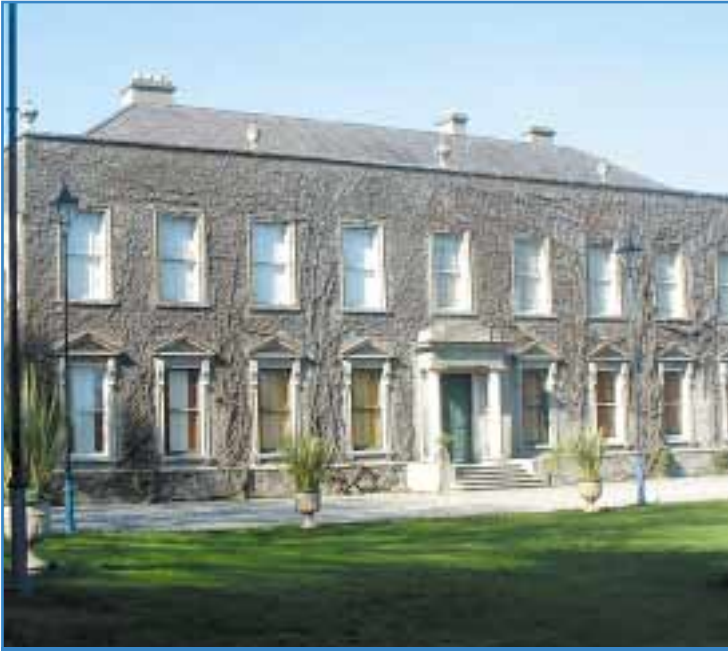
Cabinteely Park House
