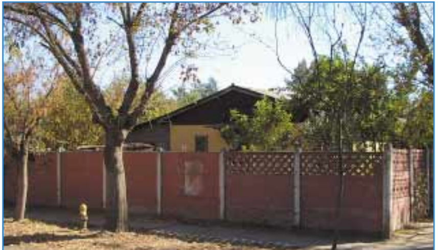
The Completed House
